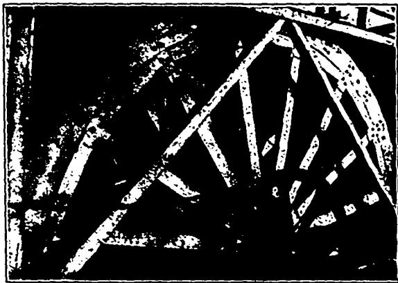
Large Water Wheel, 28 ft. diameter and 7½ ft. face, on Willow River.
