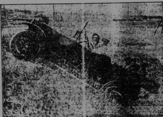
A 1916 Studebaker Four making a grade 22 feet long through deep sand at Longmont, Colo., with a start of but 78 feet. The gasoline tank of the Studebakers being in the cowl makes certain a positive feed for an ascent of such steepness.
