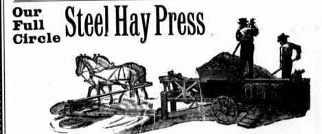
Makes two strokes of plunger for each complete turn of horses, making bales 17 in. x 22 in., and any length desired. In ordinary hay can press from ten to fifteen tons per ten hours. Absolutely the best Press on the market. We put the hind wheels five inches wide when desired.
