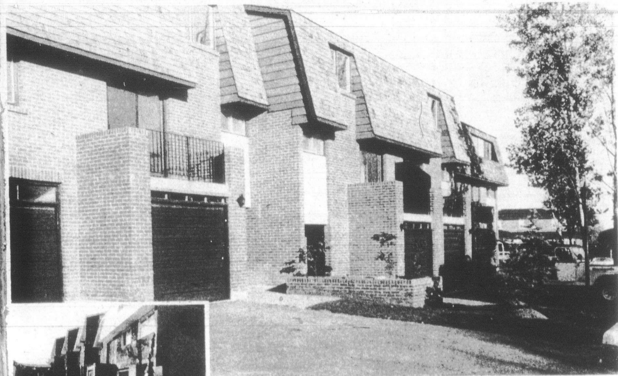
Ontim Investments Ltd. is completing the last 35 units in the 61-unit phase one Green Park Estate development. Earlier, Ontim had told council it couldn't complete the units because of poor sales. The city turned down an Ontim request to have the development split into two separate condominium communities.
