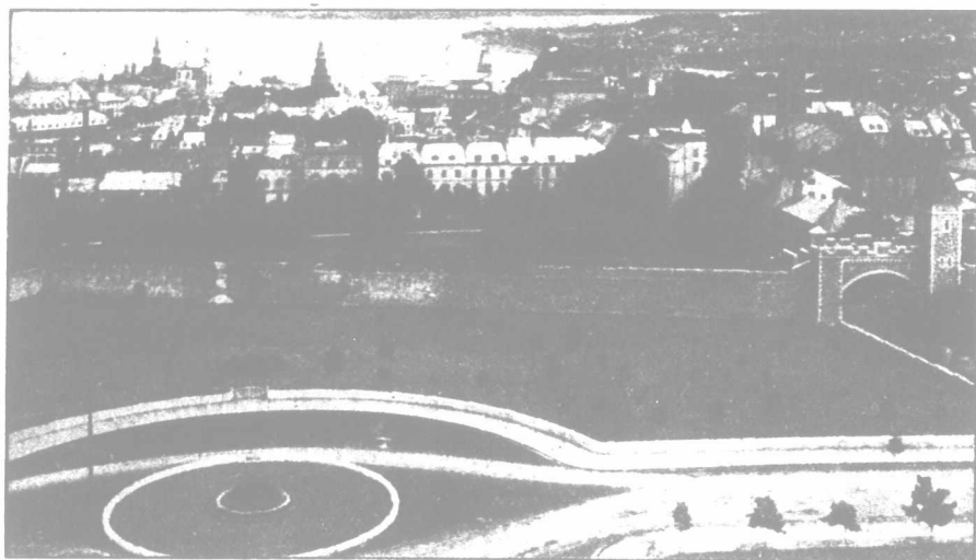
View from Parliament Buildings, Quebec, 1908, showing the walls and Kent Gate.
