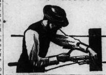
With this instrument the person stretching the wire can nail it to the post from which he is stretching without assistance.
