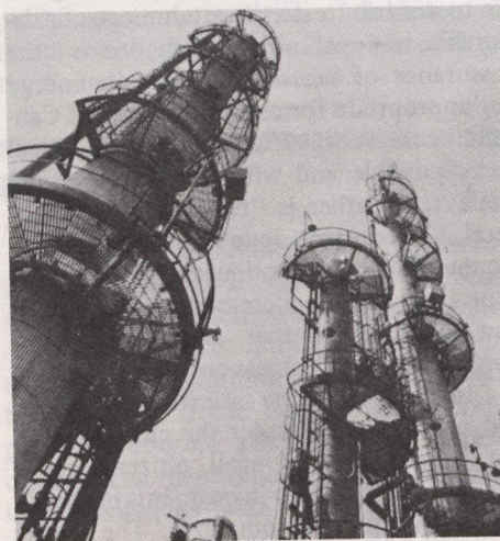
Petroleum in mist form is distilled in a “fractionating tower”.
