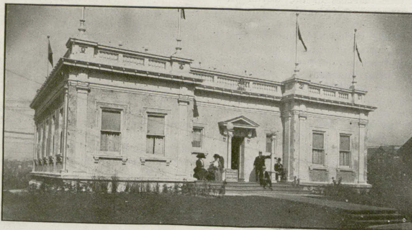
MASONIC AND EASTERN STAR REST ROOM, A-Y-P. E.
