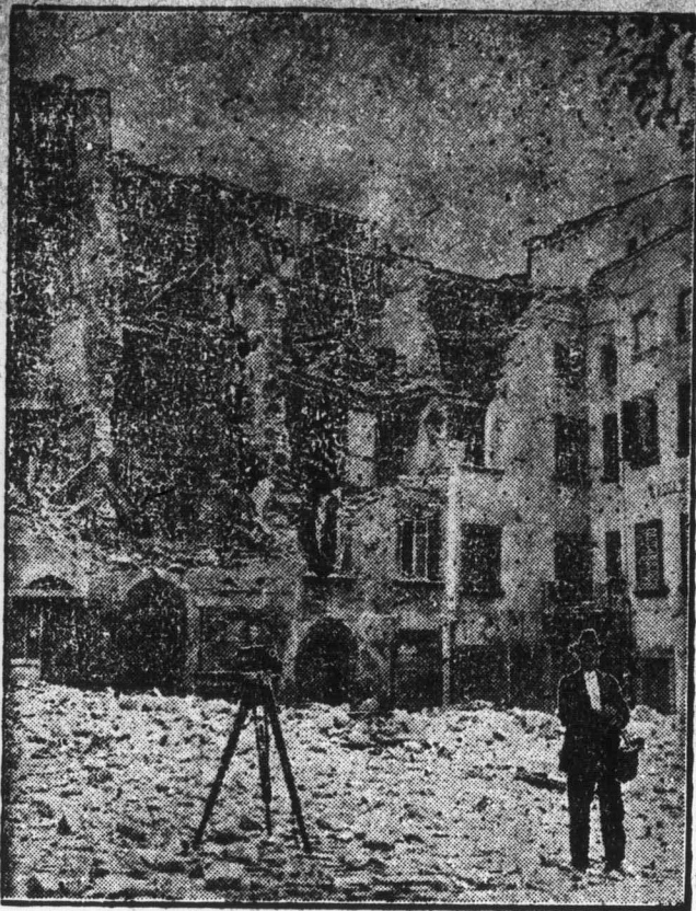
FIRST PICTURE OF DESTRUCTION CAUSED BY EARTHQUAKE IN ITALY.
