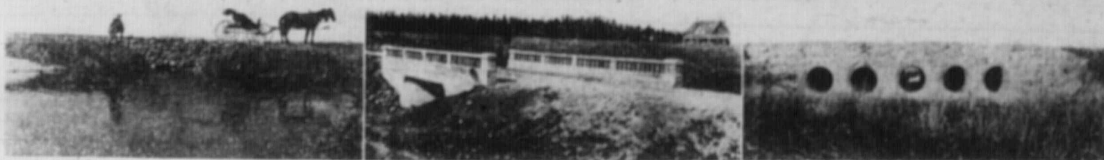
Some of the Bridges and Culverts that Wallace is Building for Posterity. These Structures will be giving service when the history of the Millennium is being written. Double 24 inch Pipe Culvert at Capacity A 14 foot Bridge with Macadam Concrete Railing A Battery of Five 24 inch Pipes Set in Concrete
