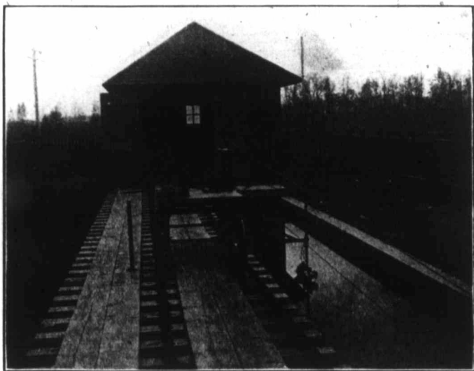
View showing car house and platform at end of tank from which to attach meter to car.
