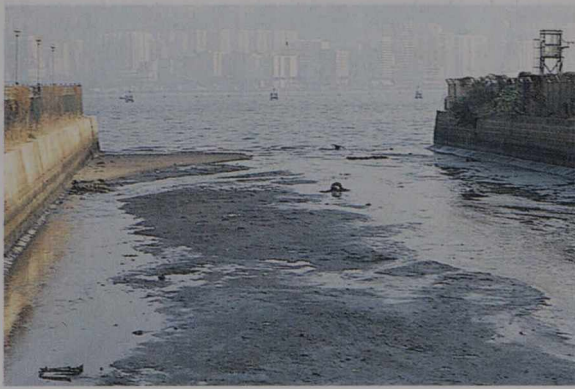
Evidence of the work that needs to be done
