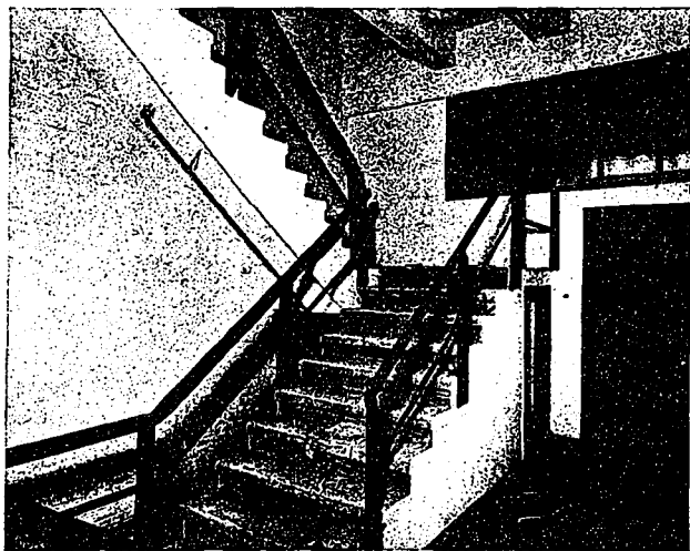
Fig. 10—VIEW OF FIREPROOF STAIRWAY, OGILVIE BUILDING, TORONTO, SHOWING THE SOLID CONCRETE TREADS AND IRON HANDRAIL. IN THE BACKGROUND TO THE RIGHT MAY BE SEEN ONE OF THE WALLS ENCLOSING THE PASSENGER ELEVATOR SHAFT. THE WINDOW SHOWN HAS METAL SASH AND FRAME, AND IS GLAZED WITH WIRED GLASS.
