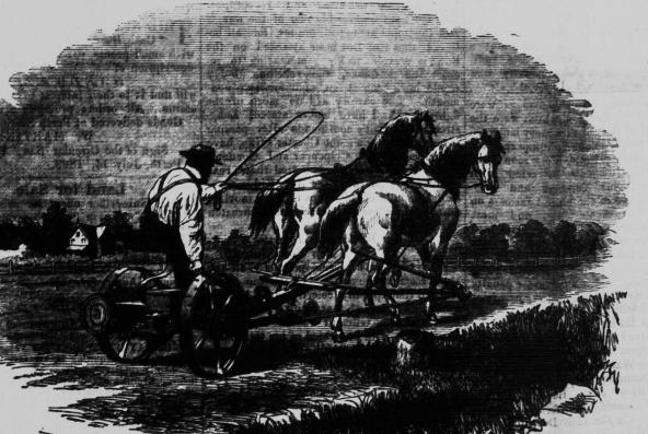
BUCKEYE MOWER WITH CUTTER BAR RAISED TO PASS AN OBSTRUCTION.
