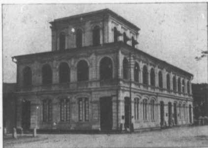
Office Building of Darley, Butler & Co. General Agents for Ceylon of the Sun Life Assurance Company of Canada.
