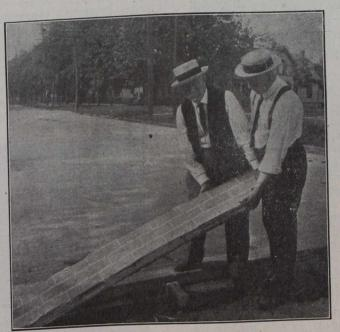
Fig. 1.—A Section of Pavement. This illustrates the perfect application of the cement filler.
