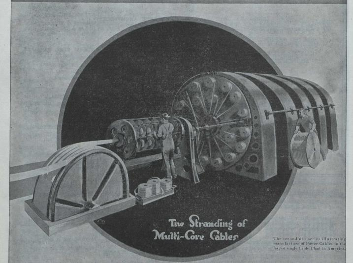
PHIS illustration shows another important process in the building of N. E. Paper Insulated Power Cables. The insulated conductors are drawn through the machine from reels located in the rear section and twisted together with jute ropes to form a circular core by the revolving motion of the outer frame.
