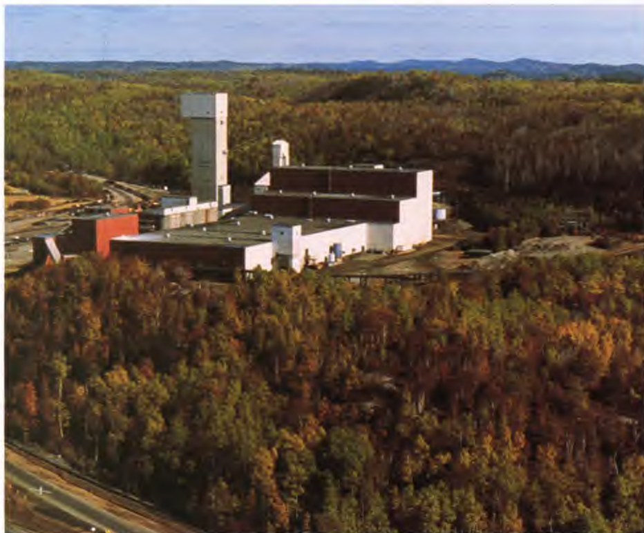
Falconbridge's Strathcona mine and mill complex in Onaping, Ontario, in the Sudbury Basin.
