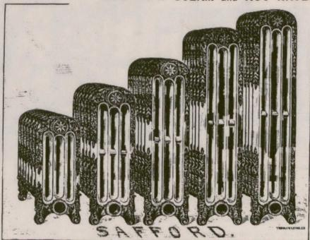
The Only Radiator made without Bolts, Packing or Washers. Cannot leak; every inch guaranteed surface. Only weigh six pounds to foot, and hold 14½ gallons of water per hundred feet of surface.
