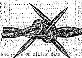
**Four-Point Barb Galvanized steel Wire Fencing.**
