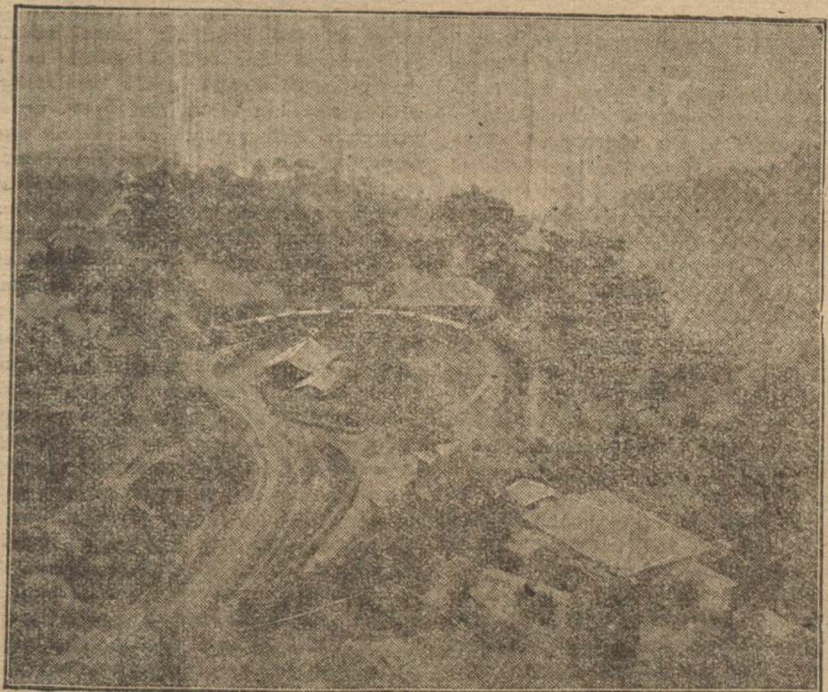
A LOOP OF THE NARROW GAUGE ROAD ON THE HIMALAYA MOUNTAINS.
