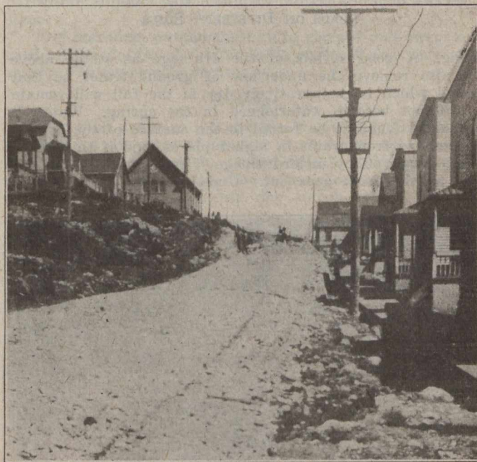
BLASTING ROCK ON A COBALT STREET WITHIN 20 FT. OF A HOUSE—NO DAMAGE DONE
