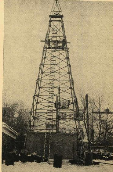
The purpose of this derrick is to enable the Dominion Observatory to drill a hole with a diamond drill 2,000 feet down to measure heat flow through the rocks of the earth. Observation: the further down you go, the hotter it is. They want to measure the rate.
