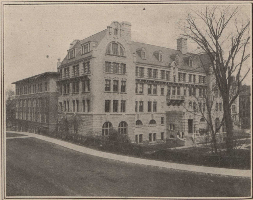
The New Macdonald Engineering Building
