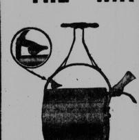
This roller can be made as heavy or as light as desired by simply putting in the right amount of water or sand. The advantage of this is obvious, for you are not handling any extra weight and for storing away it can be emptied entirely.
