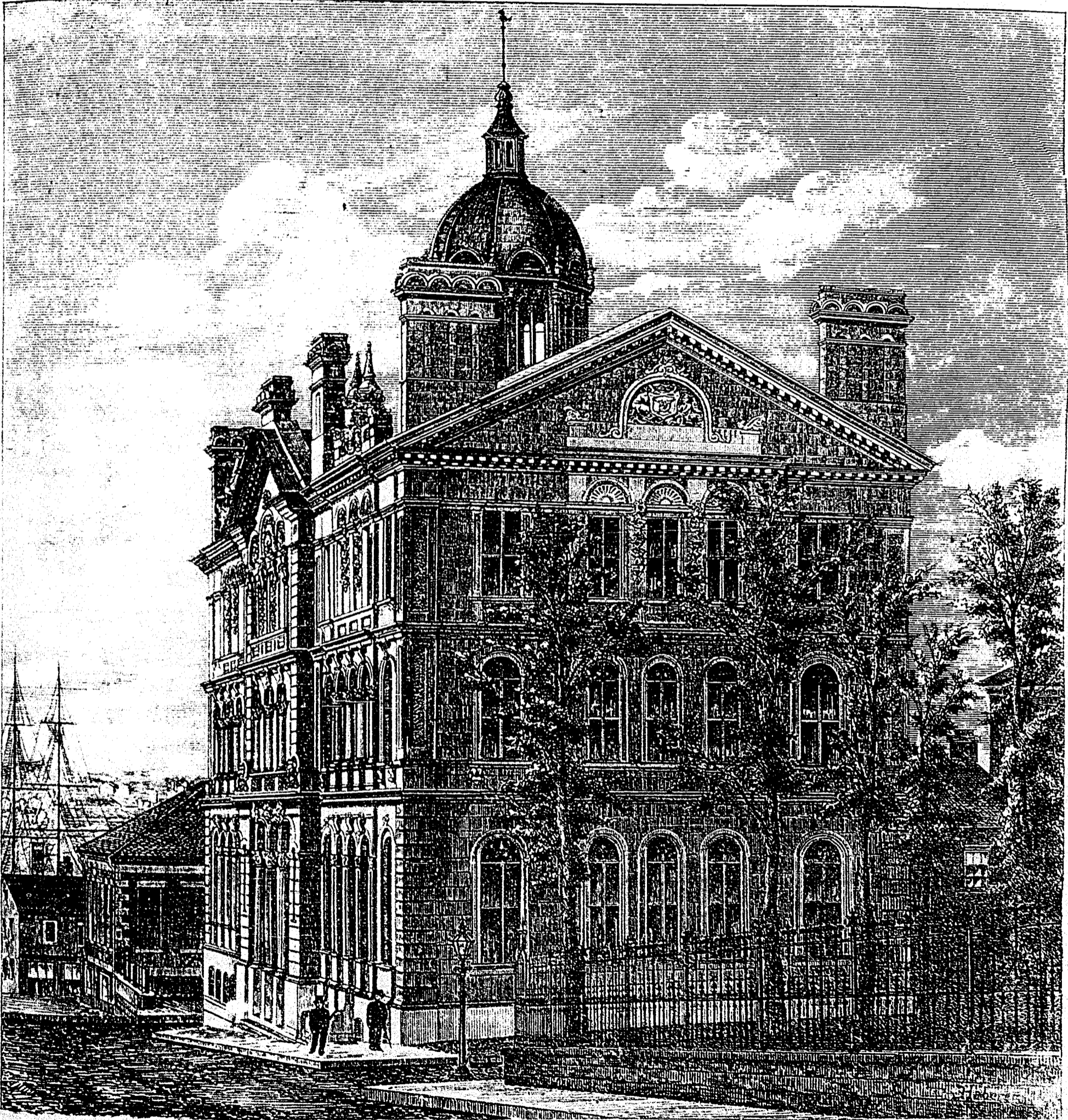
THE NEW POST OFFICE (PROVINCIAL BUILDING), HALIFAX, N. S.—SEE PAGE 354.
