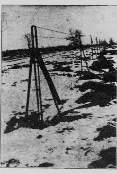
2. End, or Anchor Posts take entire strain of a wire fence. Ours
