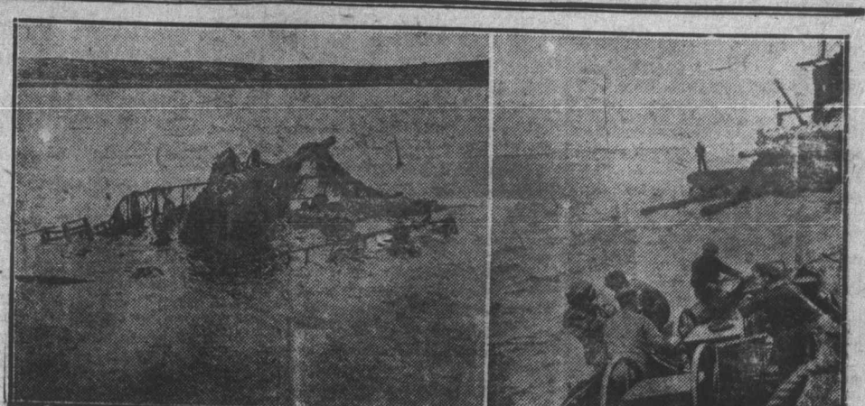
SALVING THE SUNKEN GERMAN FLEET AT SCAPA FLOW. Our photographs show a destroyer and a battleship just as they made their appearance above water. They are entangled in sea-weed and covered with rust. Note the diver about to descend.
