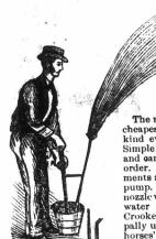
The most useful and cheapest article of the kind ever introduced. Simple in construction and cannot get out of order. Three attach-ments accompany each pump. 1st—Straight nozzle which will throw water 50 feet. 2nd— Crooked nozzle, principally used for washing horses' legs, buggies, etc. 3rd (which is rep-
