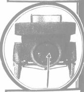
Note the compact arrangement f spare tire carrier, tail light and cense bracket.
