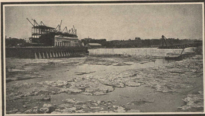
Dam, Forebay and Sluice-gates—Electrical Development Company, Niagara.
