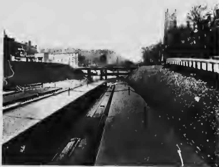
The Mount Royal Tunnel Route
