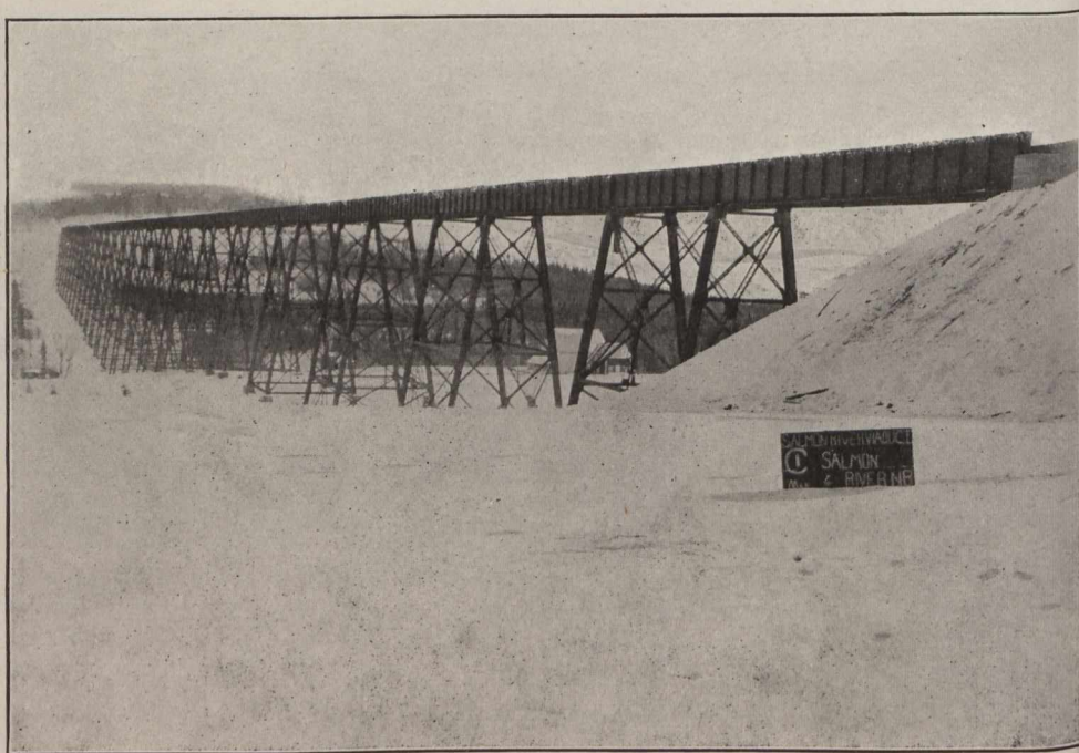
Little Salmon River Viaduct, New Brunswick. Mile 184 from Moncton. Length, 3,918 ft. Height, 200 ft. Tons Steel, 6,995.
