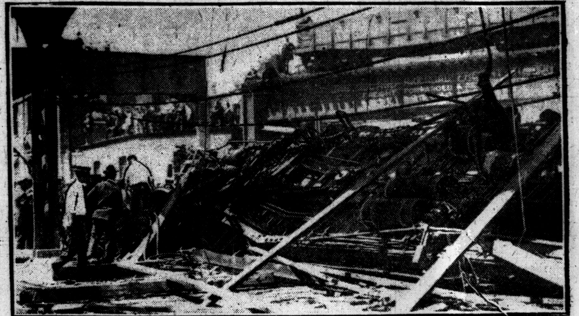
Clearing away the wreckage of the Brooklyn elevated smash where six were killed was a slow job even in New York.
