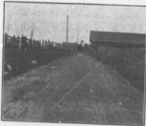
A Result of Using the Split Log Drag
