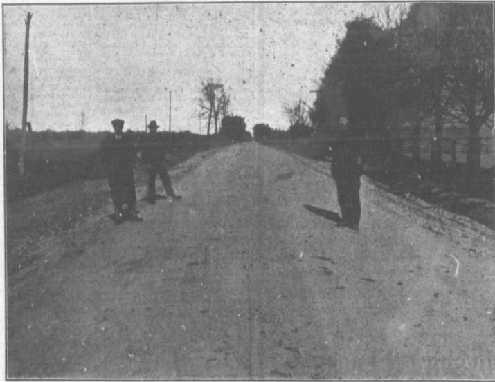
A BROKEN STONE ROAD BUILT LAST YEAR
