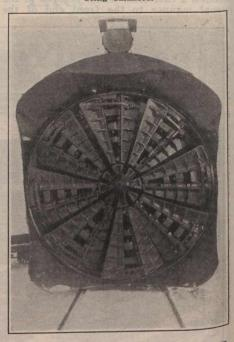
Fig. 44. Completed Wheel in Place, on C.P.R. Heavy Rotary Snow Plough.
