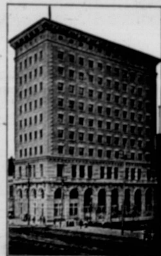
Union Bank Building, Winnipeg.
