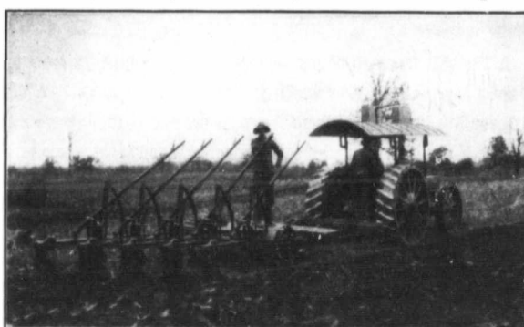
A Gould, Shapely and Muir Gas Tractor pulling a 5 bottom 14-inch Cockshutt Engine Gang in Manitoba Gumbo.
