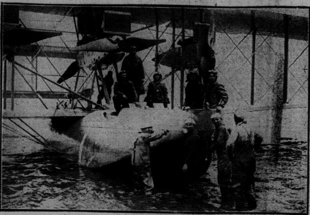
AMERICAN SEAPLANES START. ideal and issuing their orders from a foreign state. The majority of Canaphoto of one of the three planes, taken before the start, shows the type of construction. They are propelled by three sets of engines—two in front and one behind. Each carries a crew of six men.
