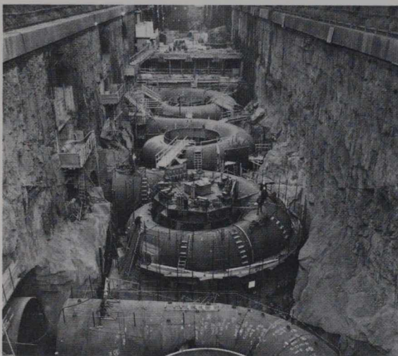
James Bay waters will turn these turbines, 140 metres underground.
