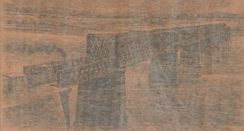
AVON RIVER BRIDGE.—WINDSOR AND ANNOVALIS RAILROAD, WINDSOR, N. S.
