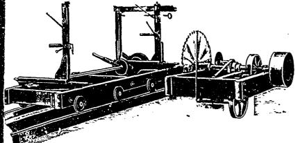
This is a Light Portable Mill for 12 to 20 H.P. It will cut from 3,000 to 8,000 ft. per day, acording to power. Can be set down ready for work in a few hours. Just the thing for light power.
