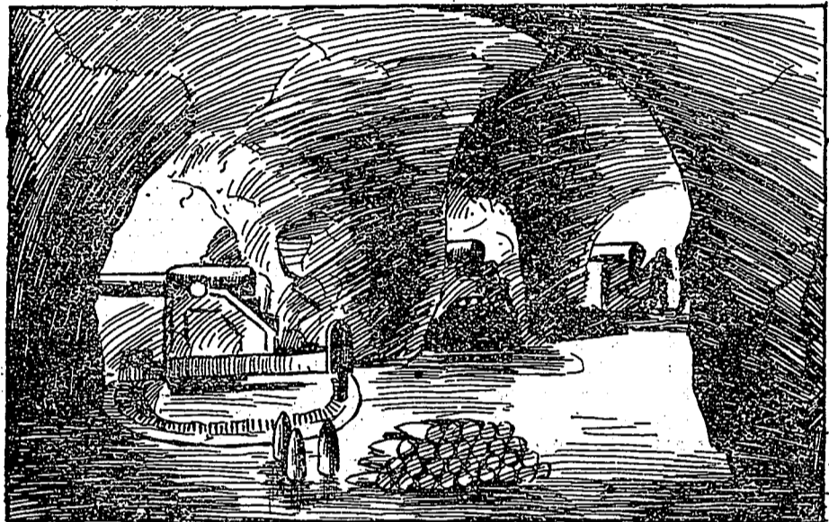
INTERIOR OF BATTERIES.
