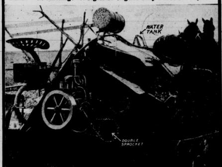
Easily and quickly attached. Our universal adjustable brackets do the trick. Anyone can run this simple 4-H. P. engine on the binder. It runs the reel and sickle, elevates, binds and delivers the grain. Team simply draws the machine. Don't overstrain your horses. Sickle continues to run when the bull wheel skids. Cut your grain when ripe. Wet weather, muddy fields have no terror where the Farm Cushman engine is used.
