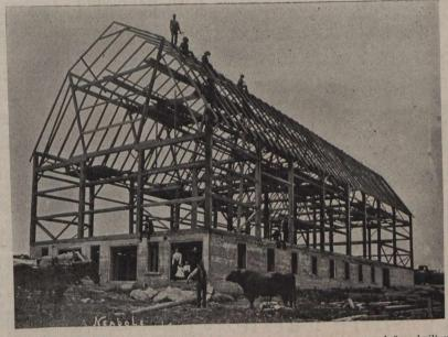
Barn of Archie Crozier, Beachburg, Ont. Size of wall, 45 x 120 ft. Wall, cistern and floor built with THOROLD CEMENT. The holes showing along the top of the wall are for ventilation. Read what Archie Crozier says about THOROLD CEMENT:
