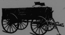
securely braced; extra heavy bottoms reinforced over the bosters. Heaver than any other bottoms made. Other special features are rivetted wheels, patent end gate and patent truss skeins that add double the carrying capacity without additional weight. Made in all sizes and handled by the
