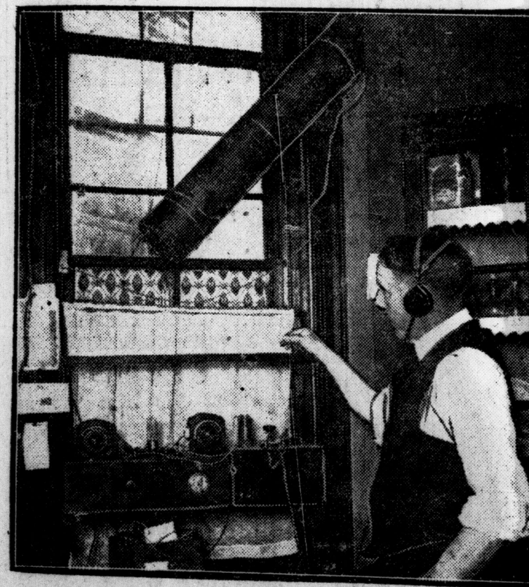
When Edward Kelly, a New York tenement dweller, was stopped from erecting an aerial on the roof, he got over his difficulty by using a few lengths of stove pipe.
