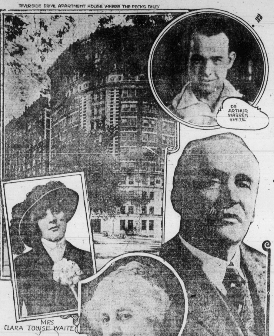
RIVERSIDE DRIVE APARTMENT HOUSE WHERE THE PECKS DIED
