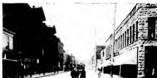
Cordova Street—Looking West.
